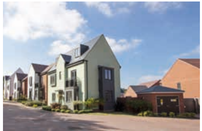
Precedent photograph illustrating integration of substations with material palettes to match neighbouring built form.
